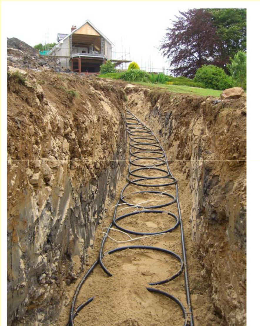
**Figure 3** Trench and SLINKY™ © GeoScience
