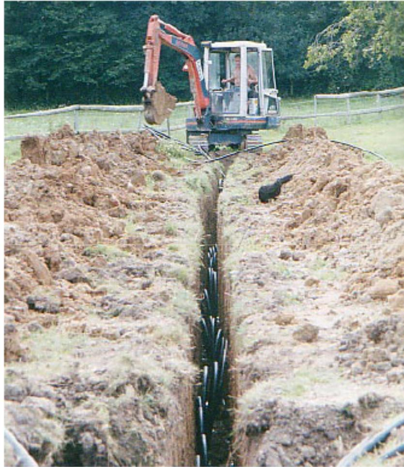
Figure 6 Installation of a vertical SUNKY ground collector © Kensa Engineering
